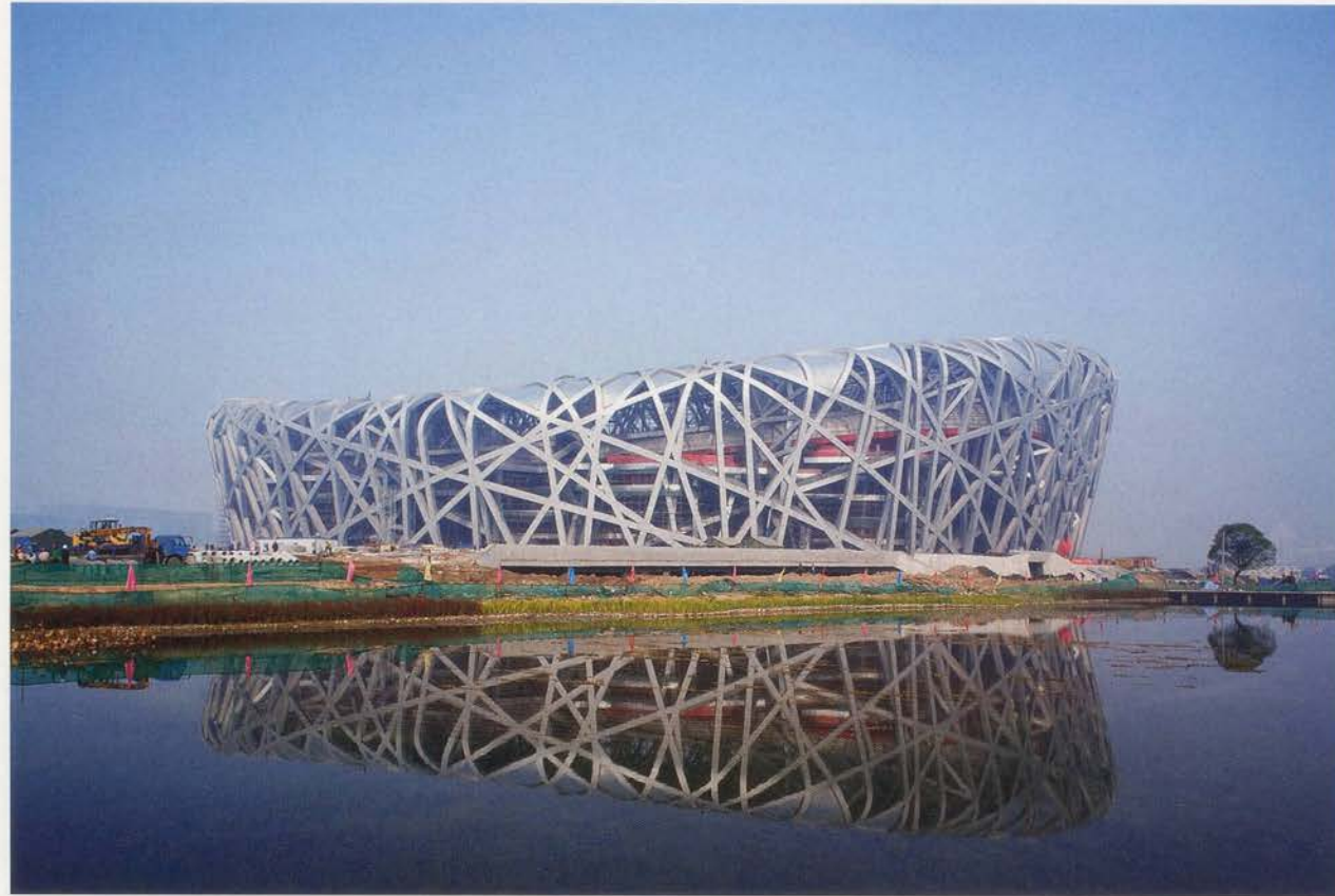
National Stadium Beijing, under construction, 2007.
